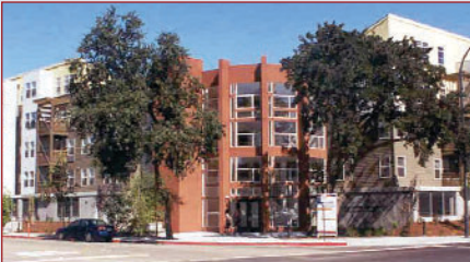
Coggins Square Pleasant Hill, Walnut Creek, CA 42 Units/Acre
