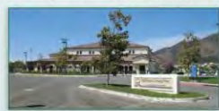
2002 Located at Borchard Road and Rancho Dos Ventos Drive, land and park improvements (including a 14,000 square foot community center) for the 28-acre Dos Ventos Community Park were dedicated to the Conejo Recreation and Park District in 2002 by the developers of the master-planned Dos Ventos Ranch community.
