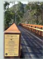
2012 The Conejo Canyons Bridge, a multi-agency cooperative effort between COSCA, the City, the District, and the County of Ventura, is dedicated. Eleven feet wide and spanning 145 feet, the bridge connects Wilwood Regional Park with Conejo Canyons Open Space.
