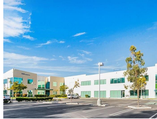
Lawrence Drive Building A
