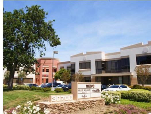
Westlake North Phase 1 Building 1
